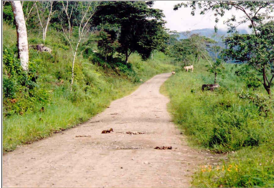
Figure 8-2: Typical Road from Mine Area to Zamora River and Junction with Amazon Highway
