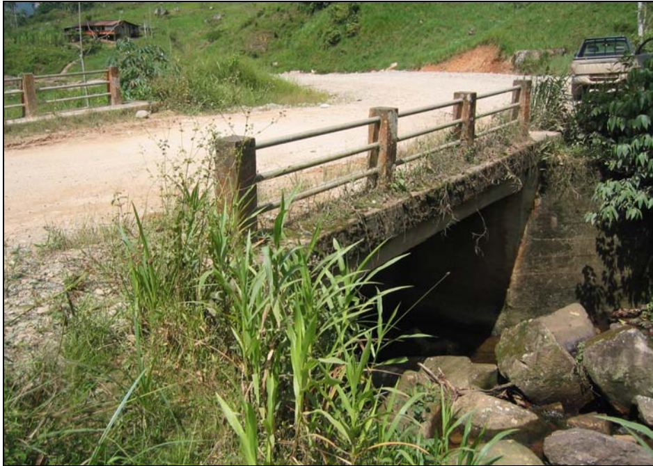
Figure 8-6: Typical Bridge Crossing for Gravelled Amazon Highway
